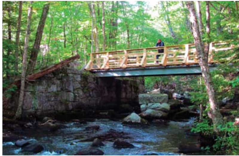
The new bridge over Nubanusit Brook in Harrisville, on the former Manchester & Keene Railroad line
