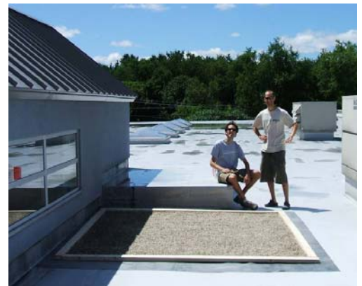
Completed nest patch. Photo by Ken Klapper.
