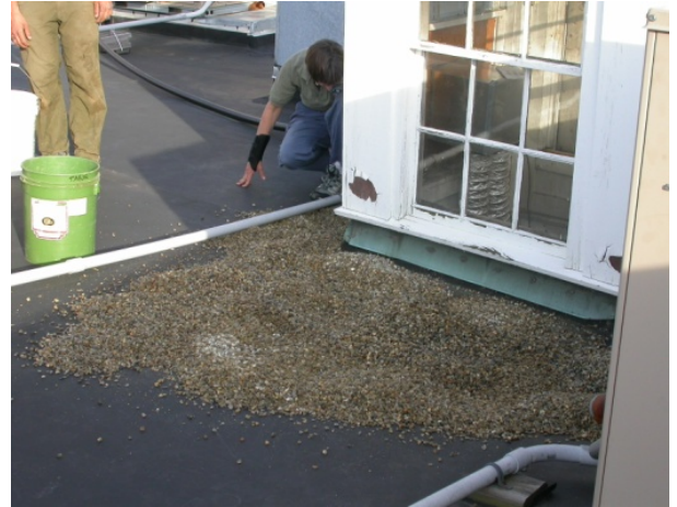
Installing a gravel patch at Sulloway & Hollis. Photo by Stephanie Parkinson.
