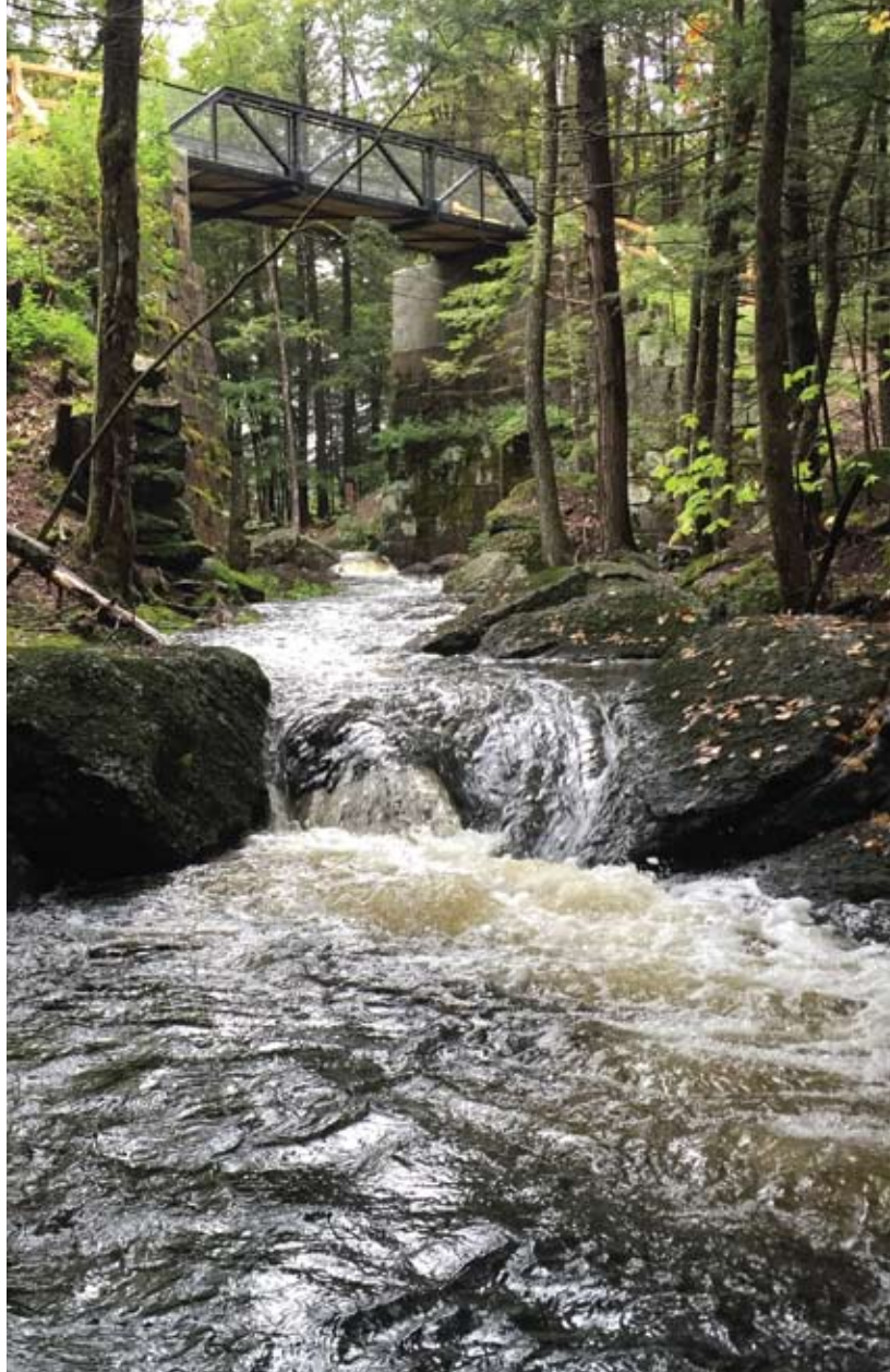
▲ Rail Trail Bridge Over Jaquith Brook photo: Jeremy Wilson
